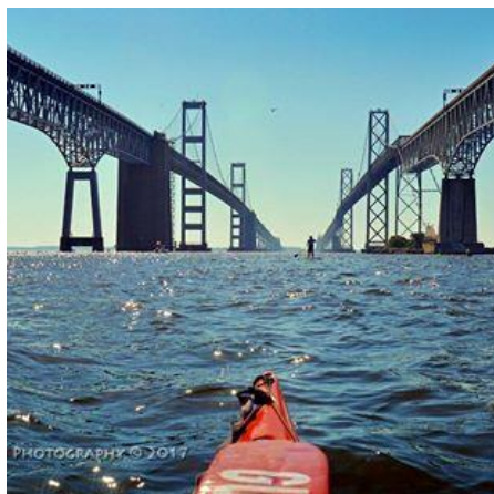
Between the two bridge spans.
